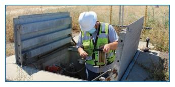
Air Force Civil Engineer Center environmental contractor, Aaron Johnson, AECOM Field Technician, inspects a groundwater extraction well at the former McClellan Air Force Base. Extracted groundwater is processed at a nearby treatment plant where clean groundwater is then returned to local creeks.
