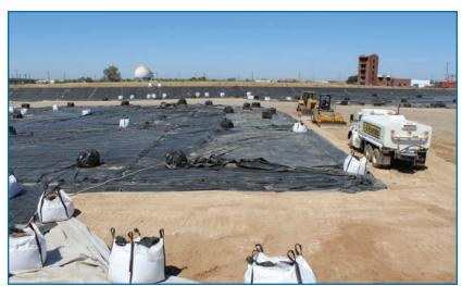
Work was also done to drain accumulated winter storm water from tarps and sump pumps at the Consolidation Unit. The CU provides a large, on-site, protected location at McClellan for excavated soils from cleanup sites during the field season which runs from April to November. In April, it began accepting soils from small excavation projects and it fully opened in May to receive more scheduled excavations from this year's field season.
